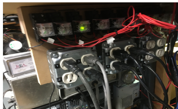
Relay and Receptacles
